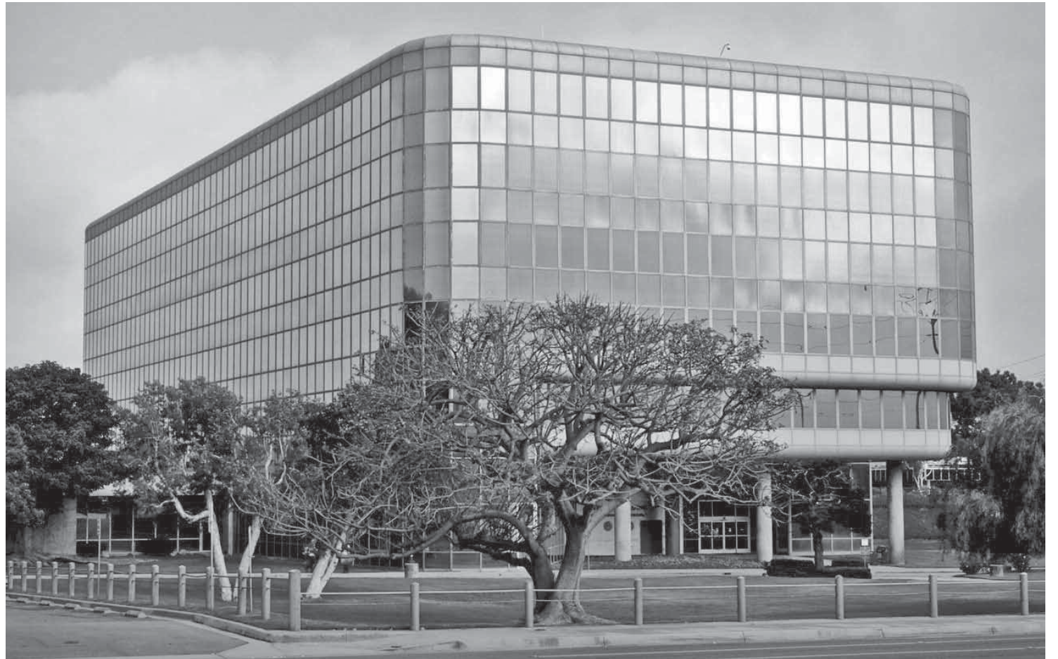
A well known and characteristic landmark in Lawndale, The Federal building at 150000 Aviation Blvd., houses the Federal Aviation Administration's West Coast Headquarters. The building was the first-designed Southern California building to have a mirrored skin. The mirrored glass skin became ubiquitous on corporate architectural designs of the 1970s and 1980s. Photo by www.christopherbarnesphotography.com.
